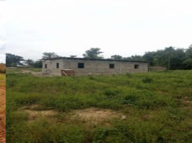
Medical Clinic Construction
