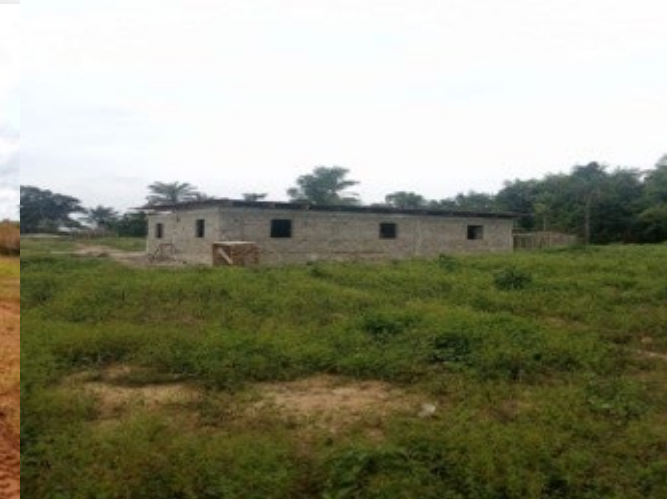
Medical Clinic Construction
