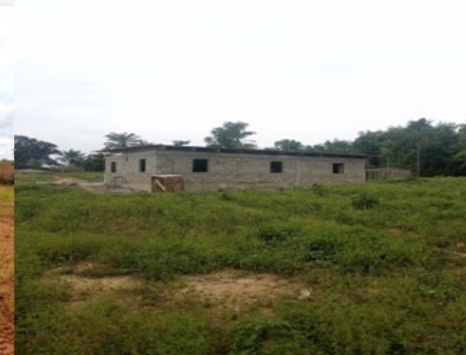
Medical Clinic Construction
