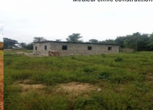
Medical clinic construction
