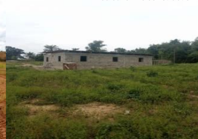
Medical clinic construction
